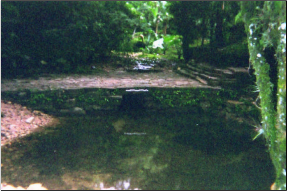
Figure 3.14 - Palenque's only fully functional bridge, OT-B1.
