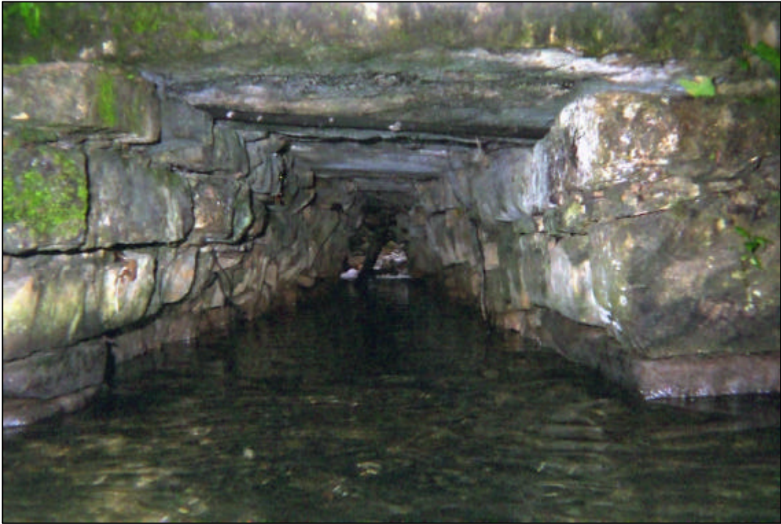
Figure 3.15 - The vaulted channel that allows for water passage beneath the bridge.
