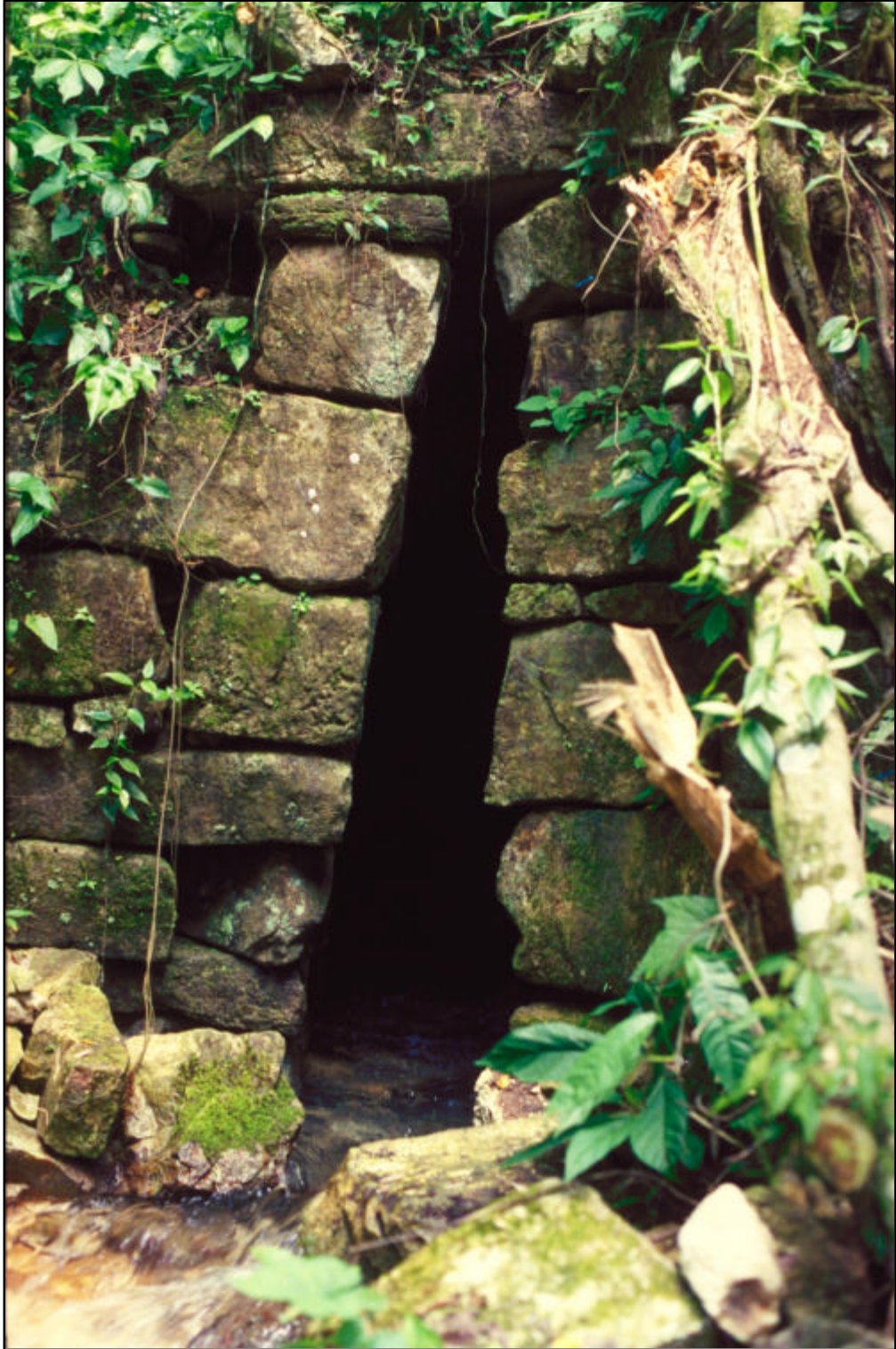
Figure 3.1 - A view of P-A1's exit.
