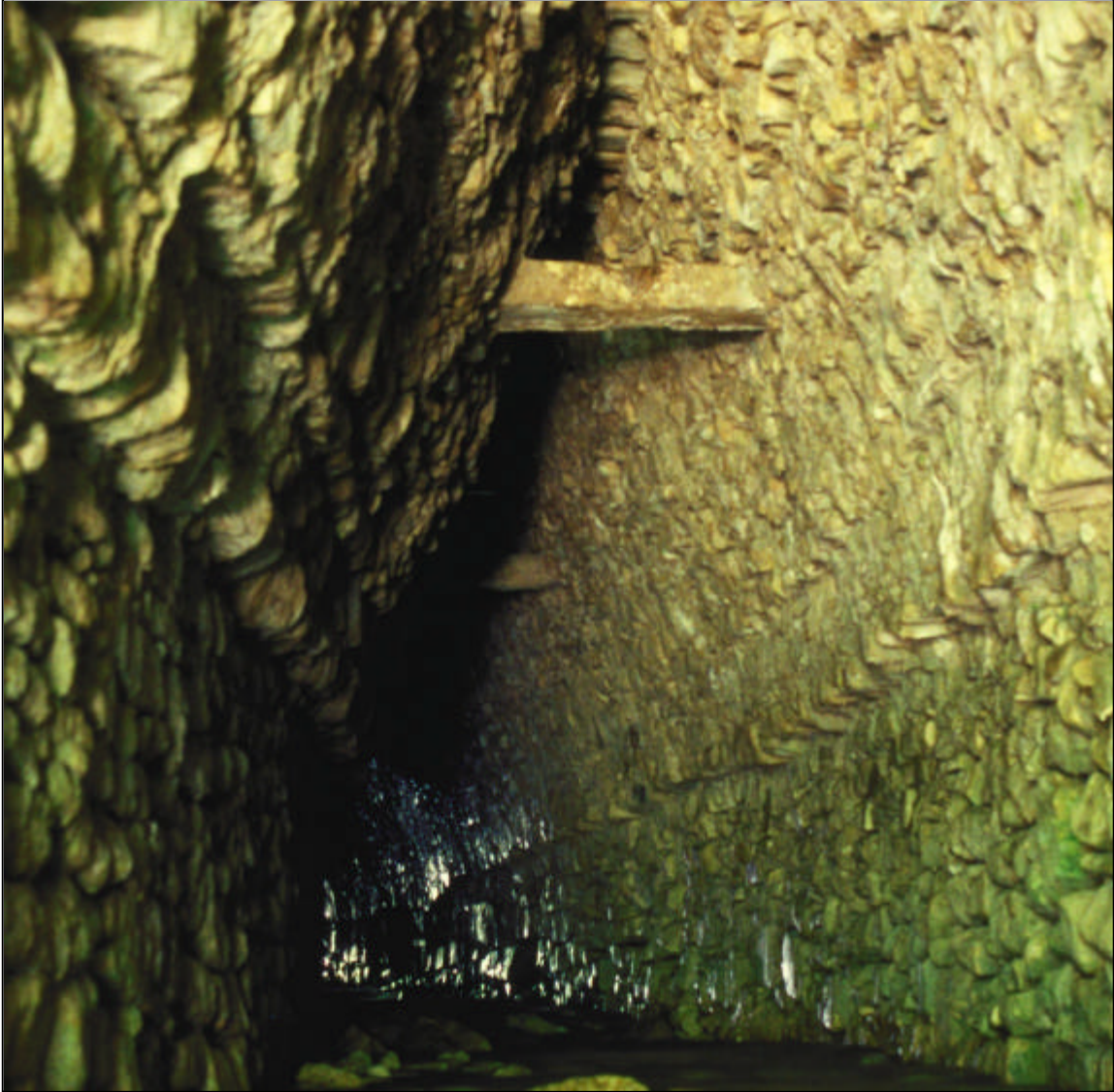
Figure 3.12 - An interior view of Palenque's best-preserved aqueduct, OT-A1. Notice the stone support beams found in the corbelled arch.
