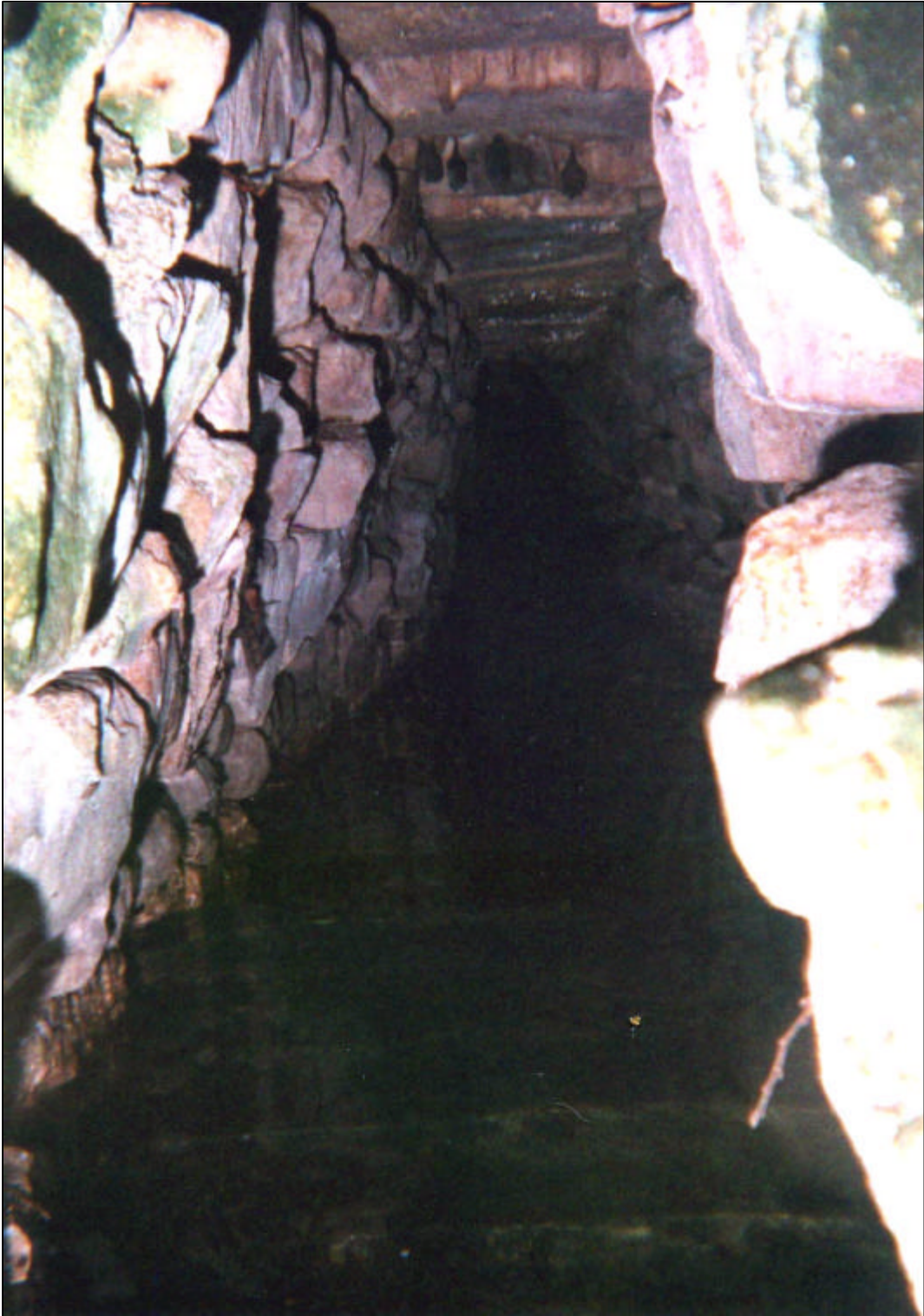
Figure 3.19 - The interior of X-A1.
