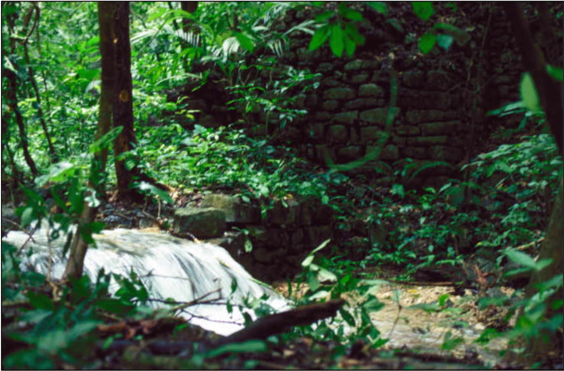
Figure 3.9 - Water flowing over MT-DM1.
